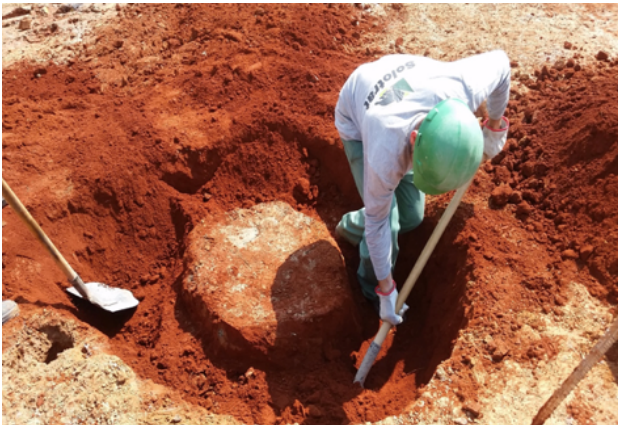
Figura 2. Coluna teste de Jet Grouting
